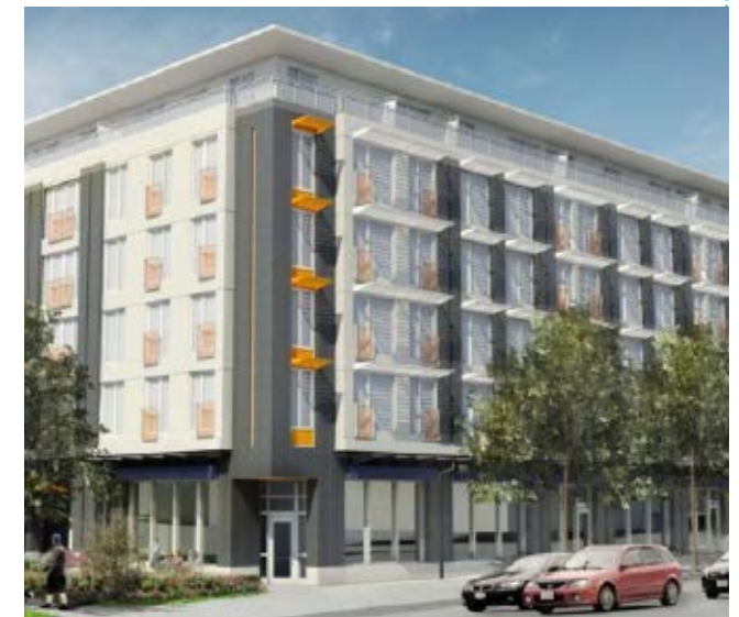
The Heights, a highly energy efficient wood-frame residential building under construction in Vancouver BC (Part 3, Step 4).
