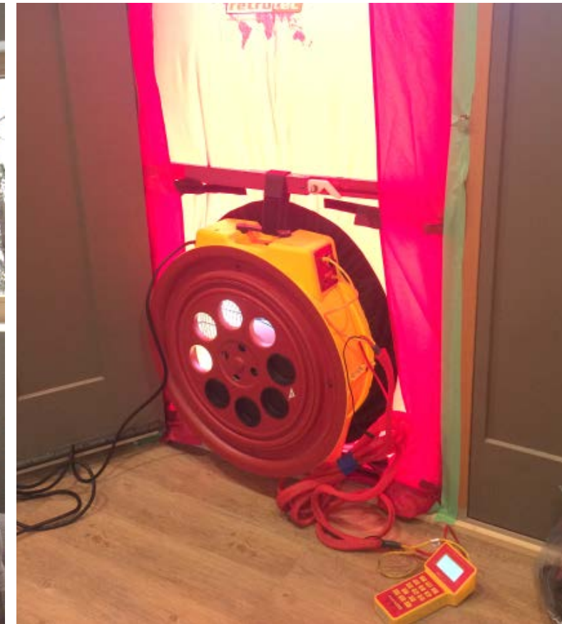
Right: Blower door testing during a builders' workshop held in Invermere BC; the home is expected to exceed EnerGuide84 (equivalent to Part 9, Step 3).
