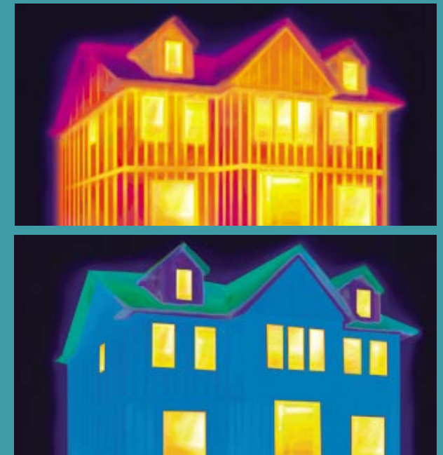
Figure 6: Example thermal images of a building demonstrating thermal bridges. Areas that are red and yellow show a lot of heat escaping through the building envelope. Blue and green areas show much less heat is escaping. Photo credit: Dow Chemical Company.
